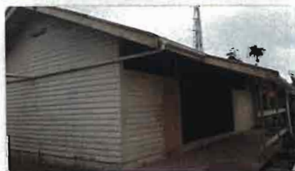
Old District Court building to be demolished
